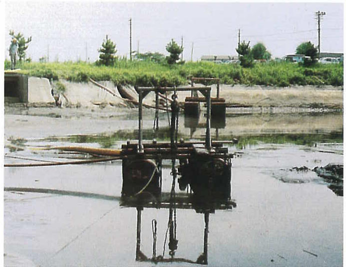
Part of the mine settling pond showing a float made from barrels suspending the pump below the liquid surface.
