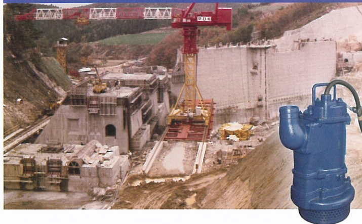
General Construction Works (V, KM, EL, EH)
